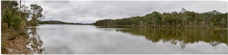
McCay Reservoir, looking down towards the dam wall and control tower. Photo: Noel Young
