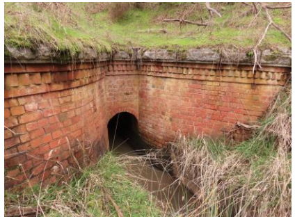
Poverty Gully Tunnel. Photo Lou Citroën
